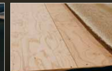
5/8" plywood floor decking
