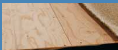
5/8" plywood floor decking
