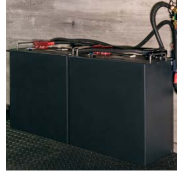
(2) 200AH 24V Lithium Batteries (which is equal to (8) 100AH 12V Lithium Batteries)*
