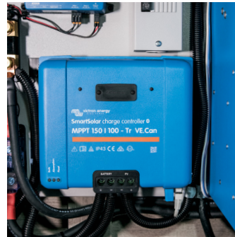
100 amp Victron MPPT Solar Charge Controller
